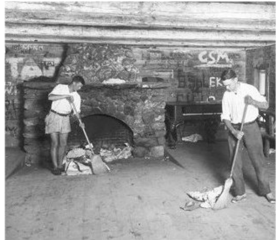
Cleaning up inside of the Lodge, 1915.
